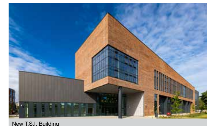
New T.S.I. Building
